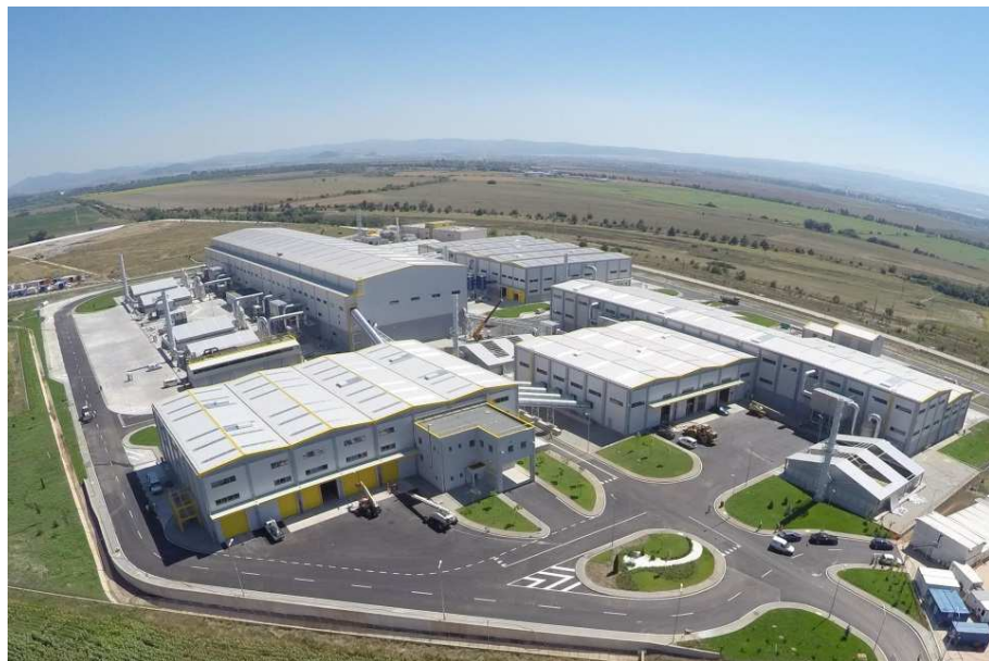
Mechanical Biological Treatment plant, Sofia, Bulgaria
